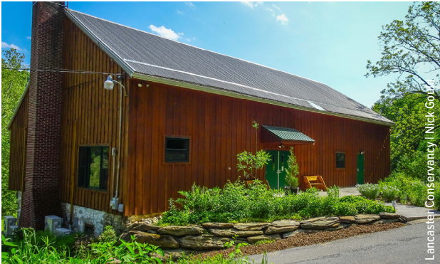
A former barn is adaptively reused as a Nature Center at Climbers Run.
