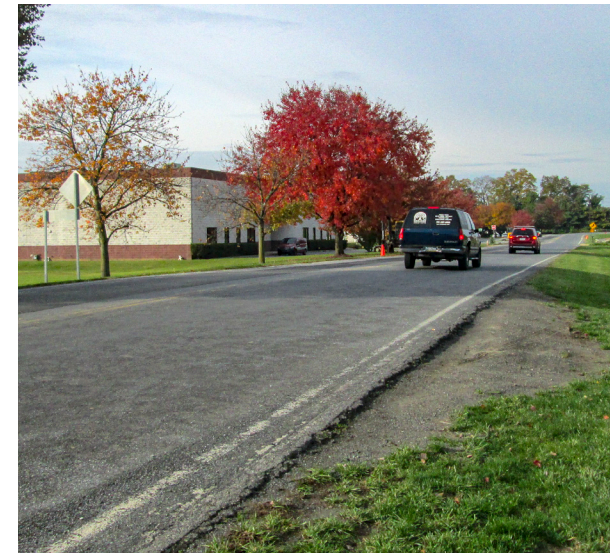
Many streets within this sector are extra wide, disconnected from surrounding development, and lack sidewalks.
