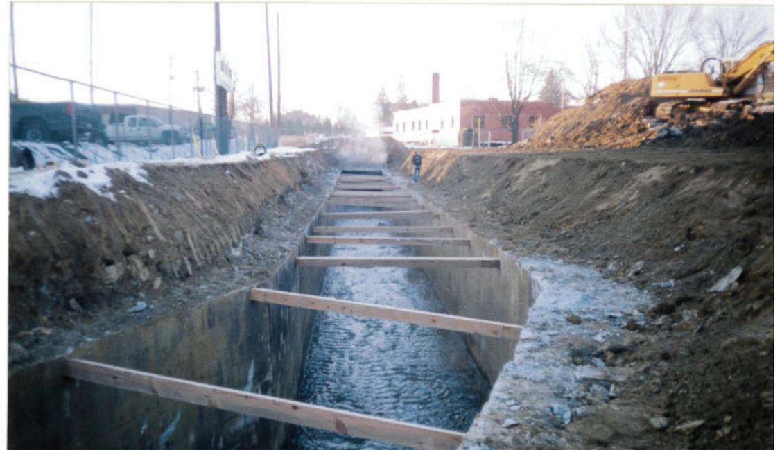
2. In 2000, Lancaster City replaced a section of the 16'-wide, 19th-century brick culvert carrying a former stream and sewage flows through Culliton Park's eastern section. Prior to its 20th-century conversion to recreational use, this site was dominated by industrial operations.
