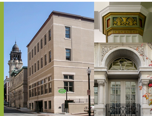
2014 Winner: Lancaster City Hall Expansion and Renovations
